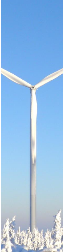
WEA wind turbines
